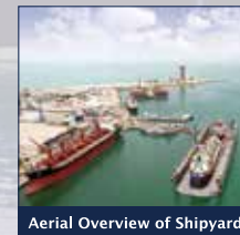
Aerial Overview of Shipyards
