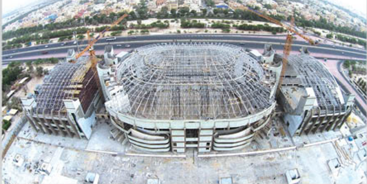
Space frame works in Sheikh Saad Al- Abdulla Sport Complex
